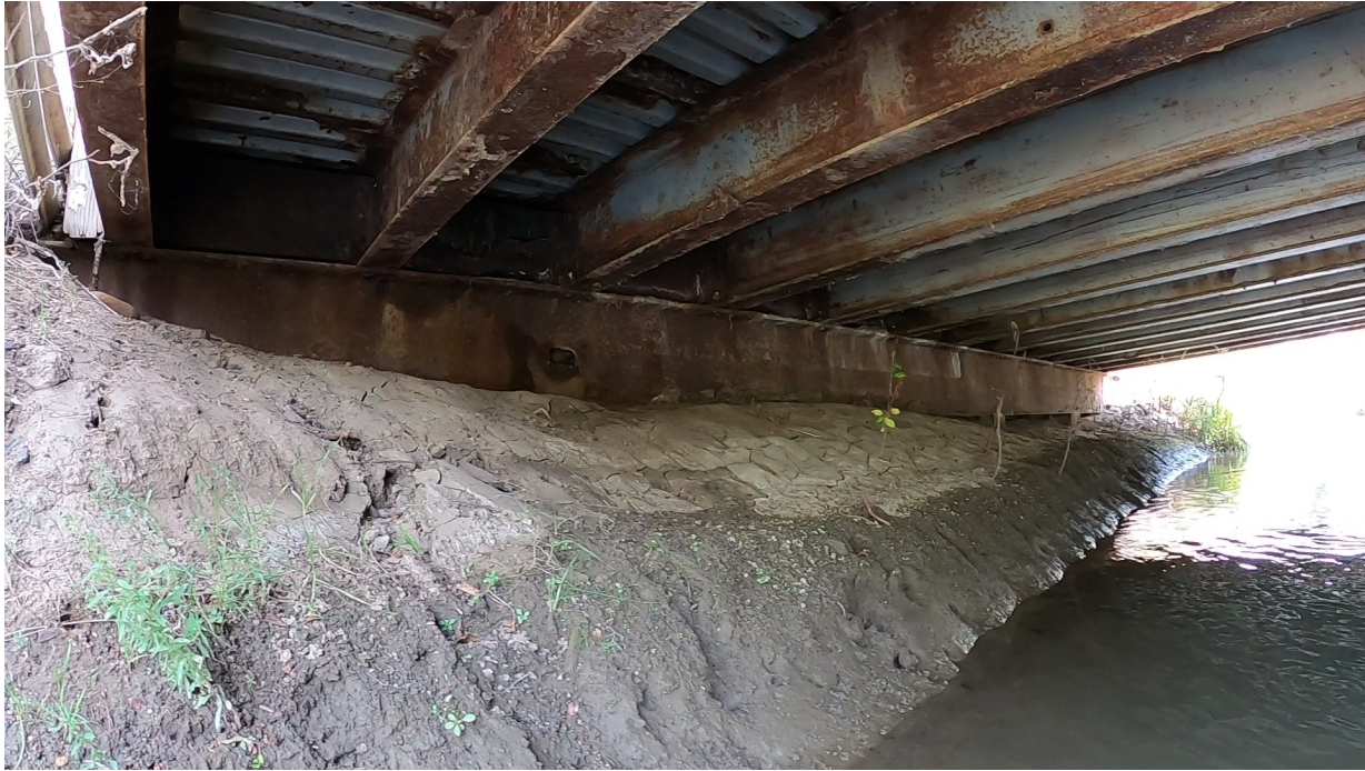
Picture 2 - Pier, Deck, Girders
