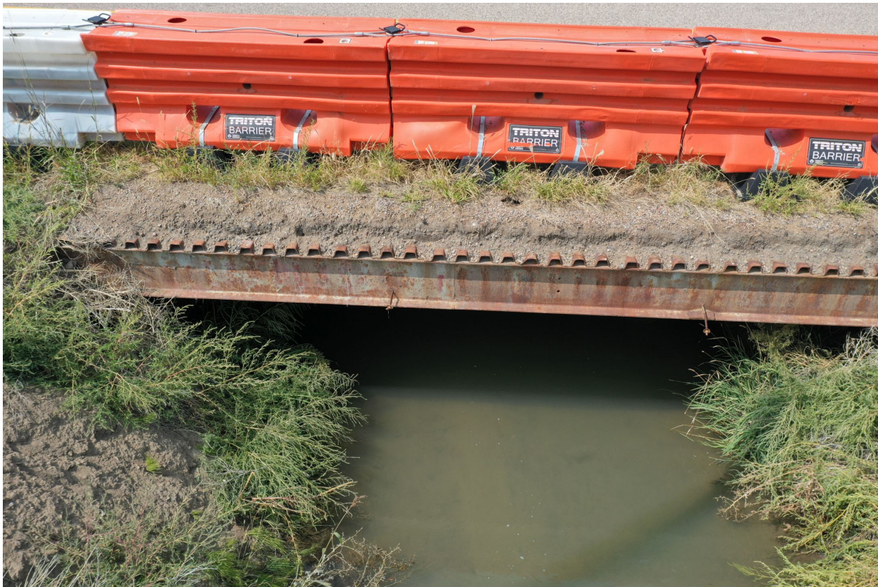
Picture 1 - Bridge P-19-G_Minor
