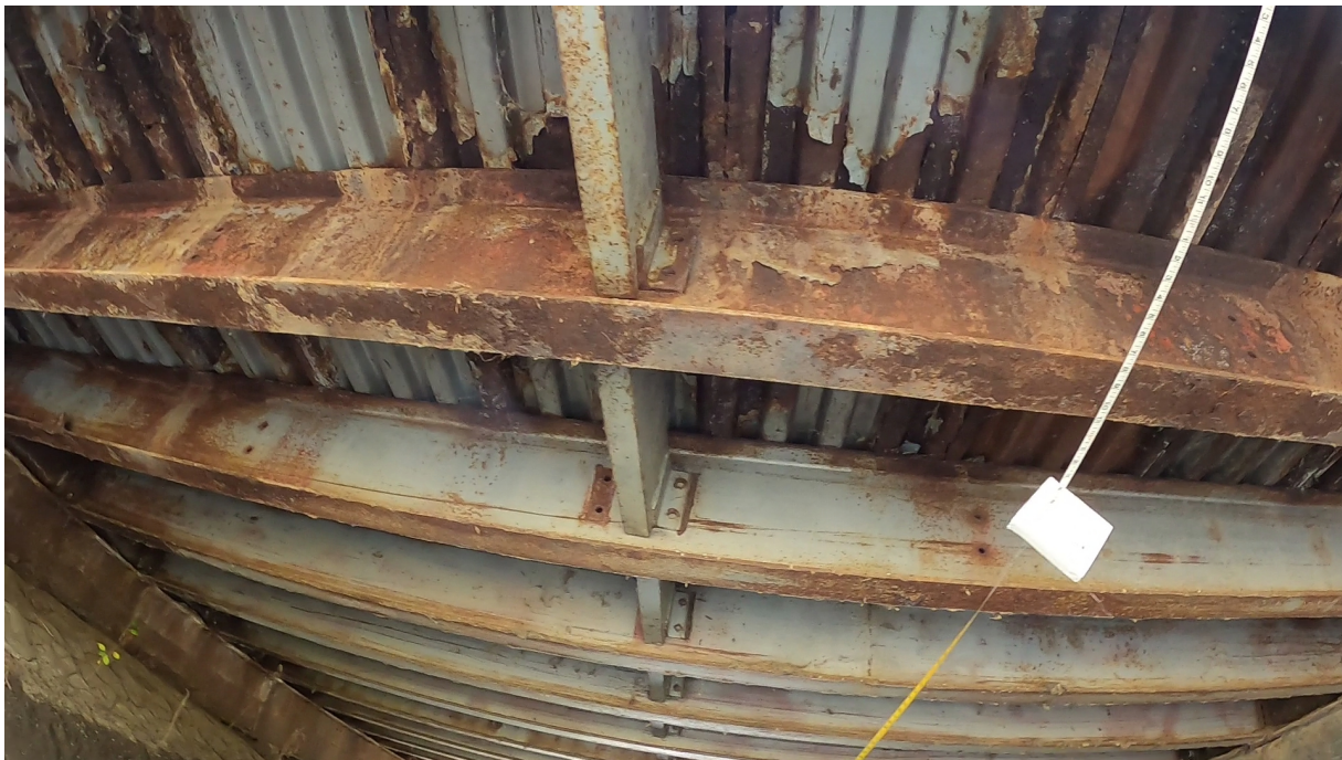
Picture 3 – Corrosion
